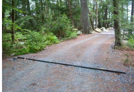
A rubber razor on a well-maintained camp road helps divert rainfall into ditches and forested areas.
