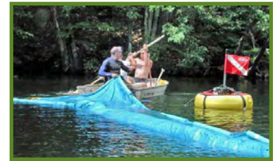
Benthic barrier installation may require divers depending on the depth of the area being managed. Photo: Peter Lowell, Lakes Environmental Association.
