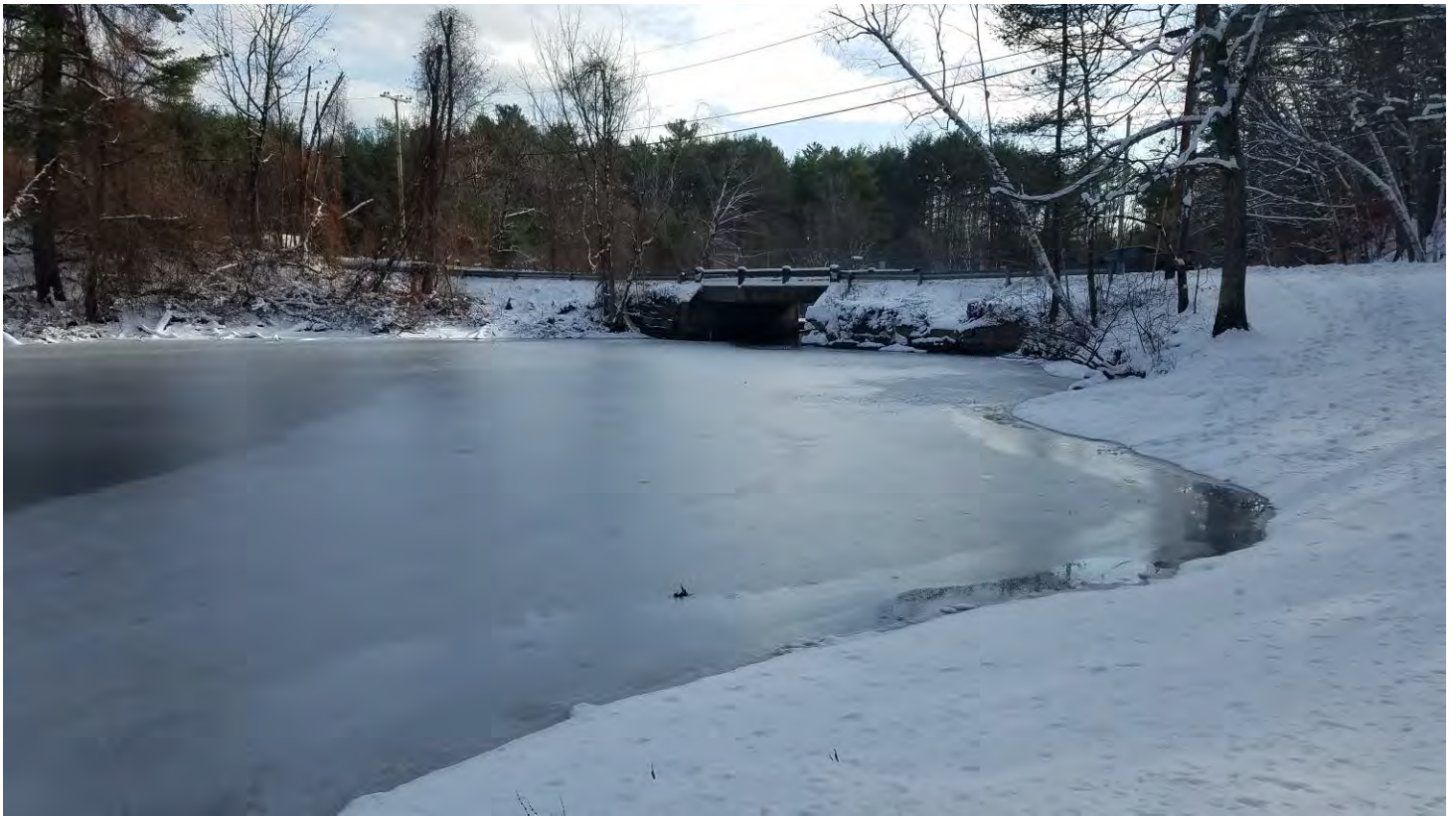
PHOTO 3: MILL STREET BRIDGE UPSTREAM OF DAM.
