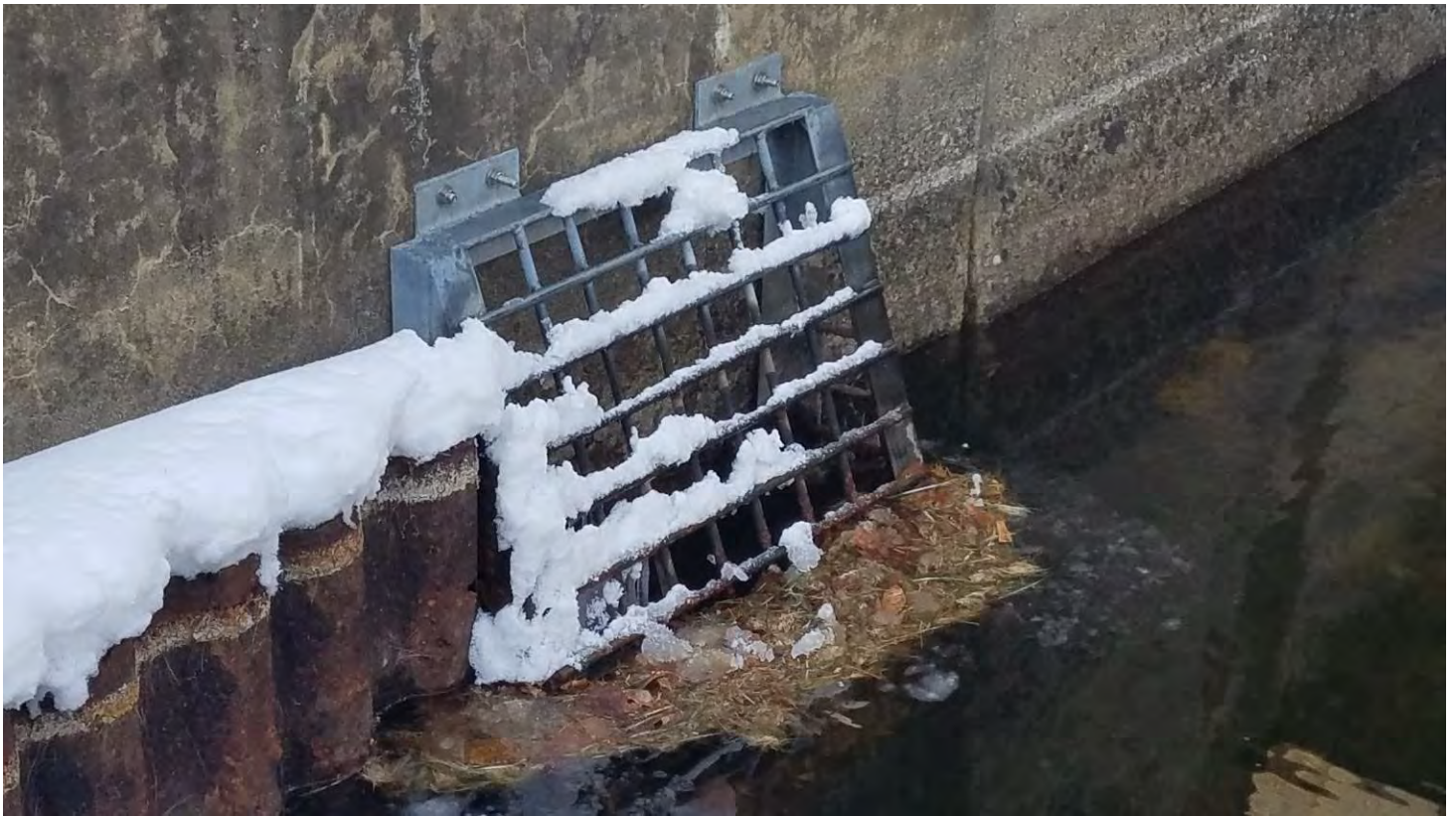
PHOTO 5: FISHWAY INTAKE GRATE.
