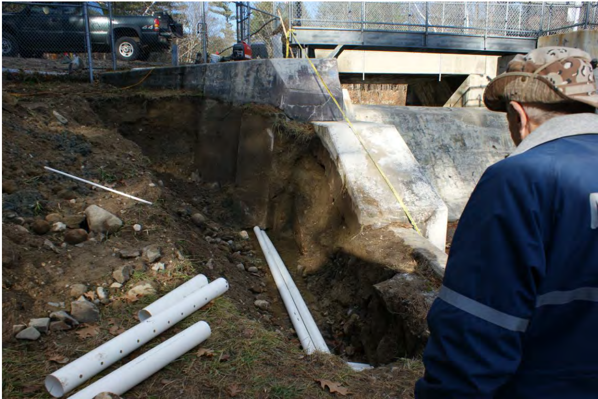
PHOTO 29: REPAIR IN 2011 DOWNSTREAM OF RIGHT ABUTMENT CUTOFF WALL.
