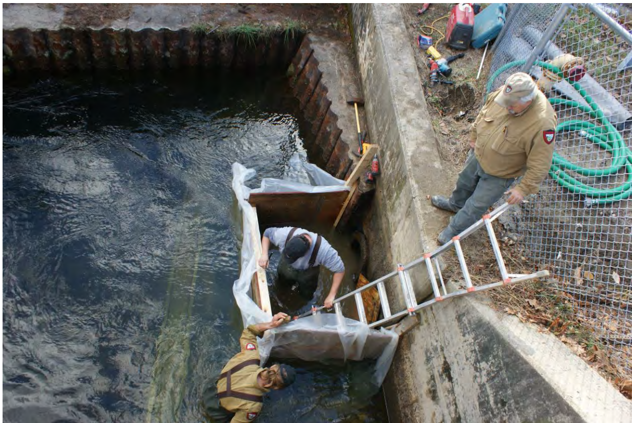
PHOTO 6: FISHWAY INTAKE DURING REPAIRS IN 2011.
