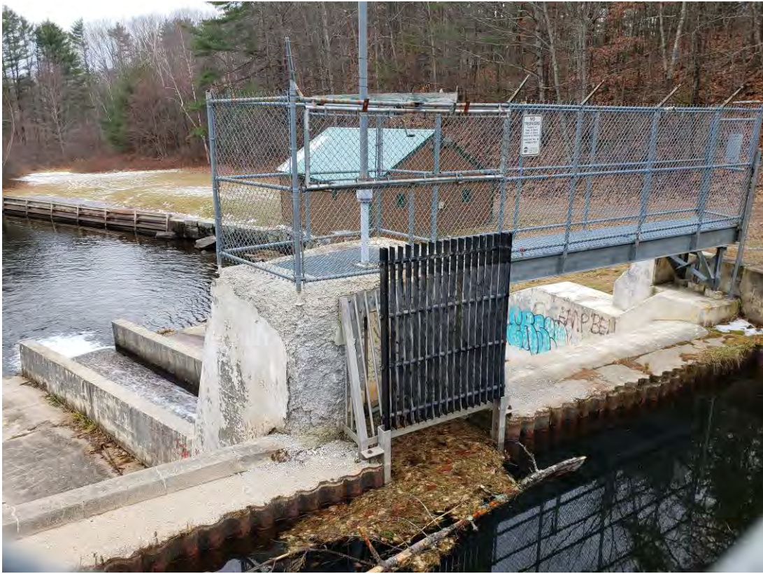
PHOTO 15: 2 FT THICK CONCRETE AND STEEL PILING.
