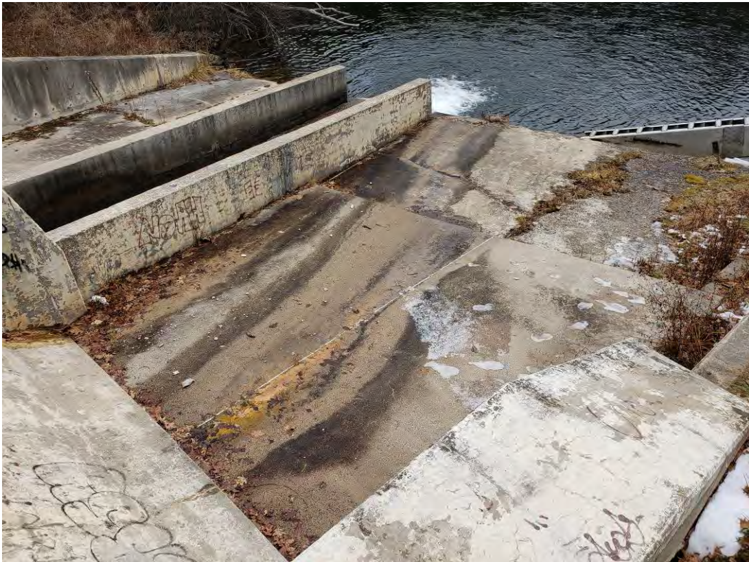
PHOTO 31: APRON DOWNSTREAM OF RIGHT OVERFLOW SPILLWAY.
