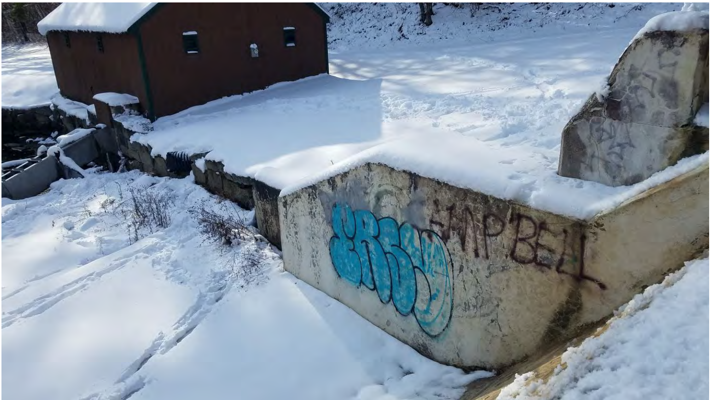
PHOTO 25: RIGHT ABUTMENT RETAINING WALL DOWNSTREAM OF DAM.
