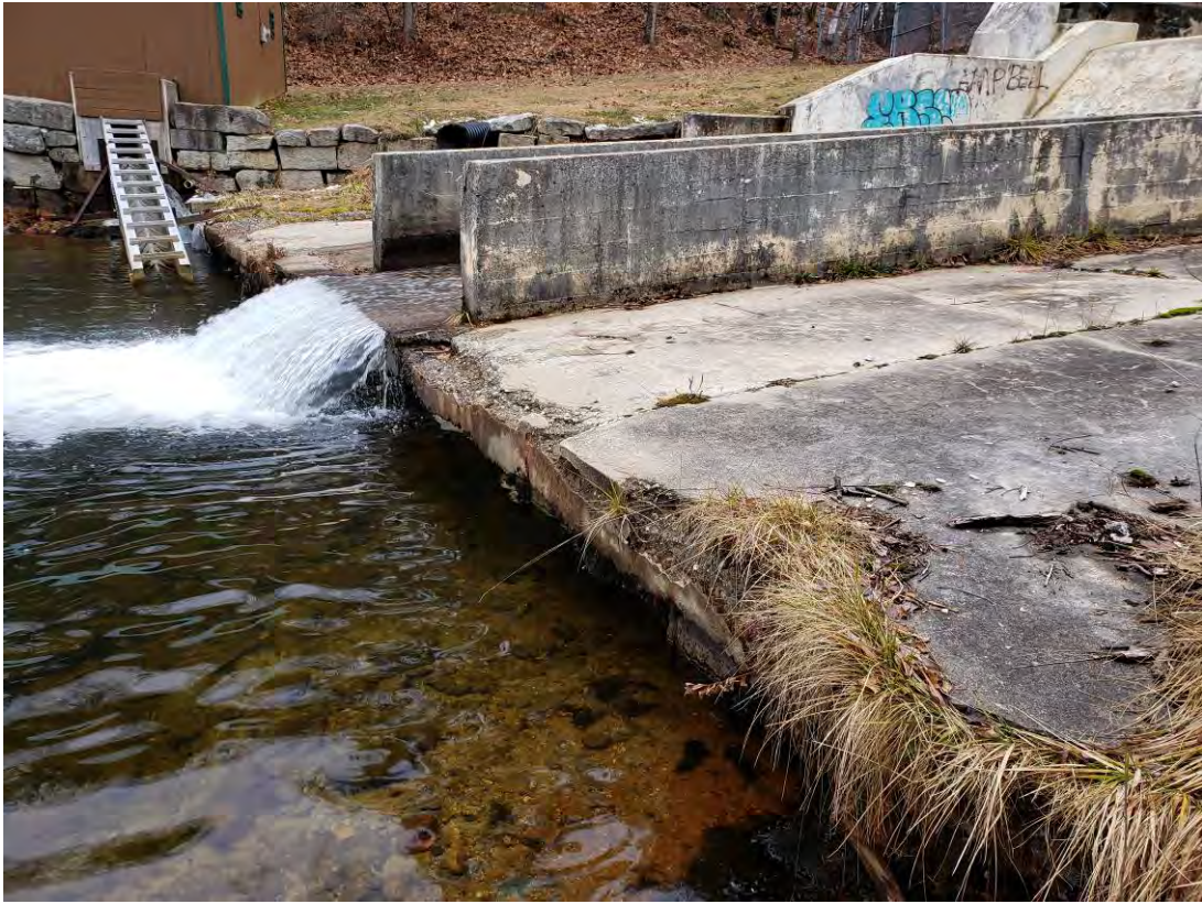
PHOTO 33: DOWNSTREAM TOE OF SPILLWAY APRON.
