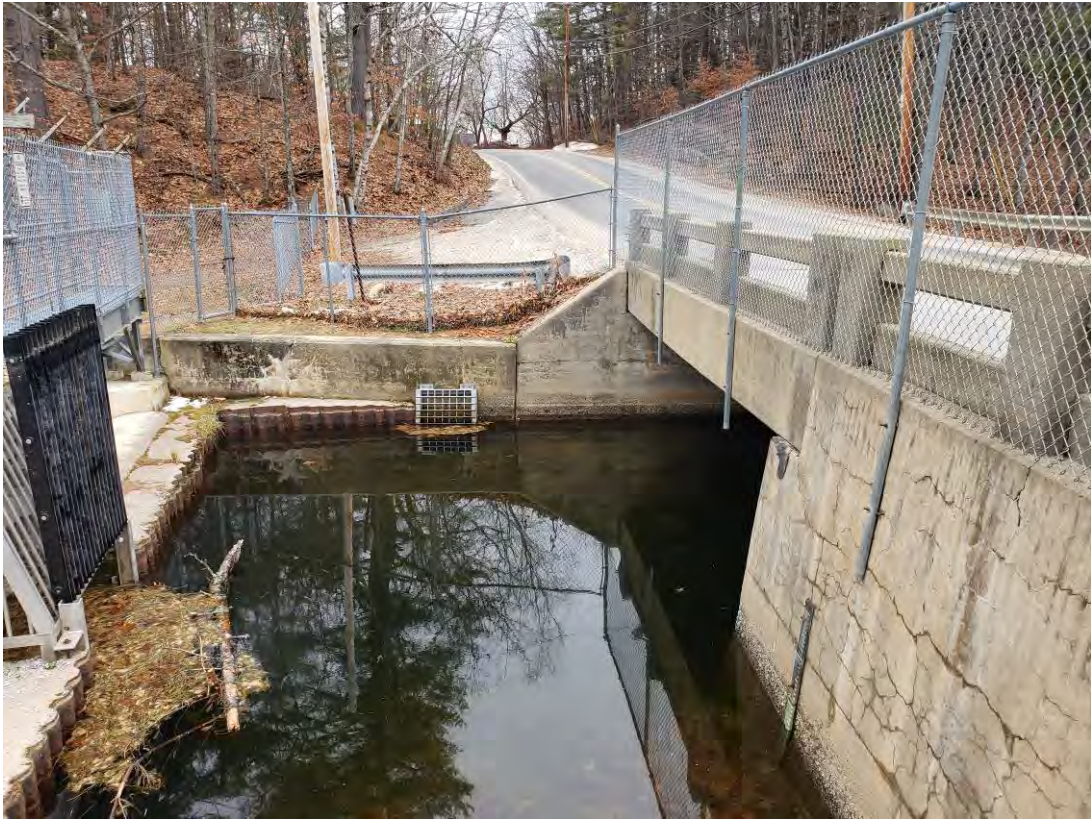
PHOTO 24: RIGHT ABUTMENT RETAINING WALL UPSTREAM OF DAM.
