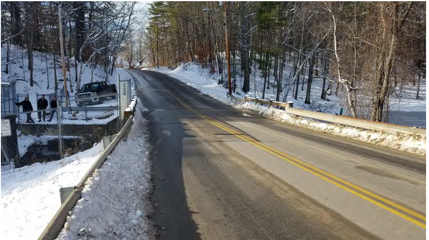
PHOTO 22: MILL STREET BRIDGE AND RIGHT ABUTMENT EMBANKMENT.
