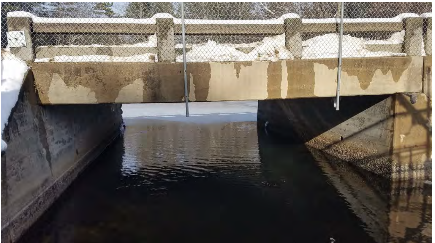
PHOTO 4: DOWNSTREAM SIDE OF MILL STREET BRIDGE.
