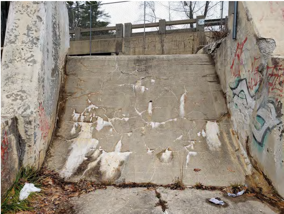
PHOTO 11: DOWNSTREAM FACE OF THE LEFT OVERFLOW SPILLWAY.
