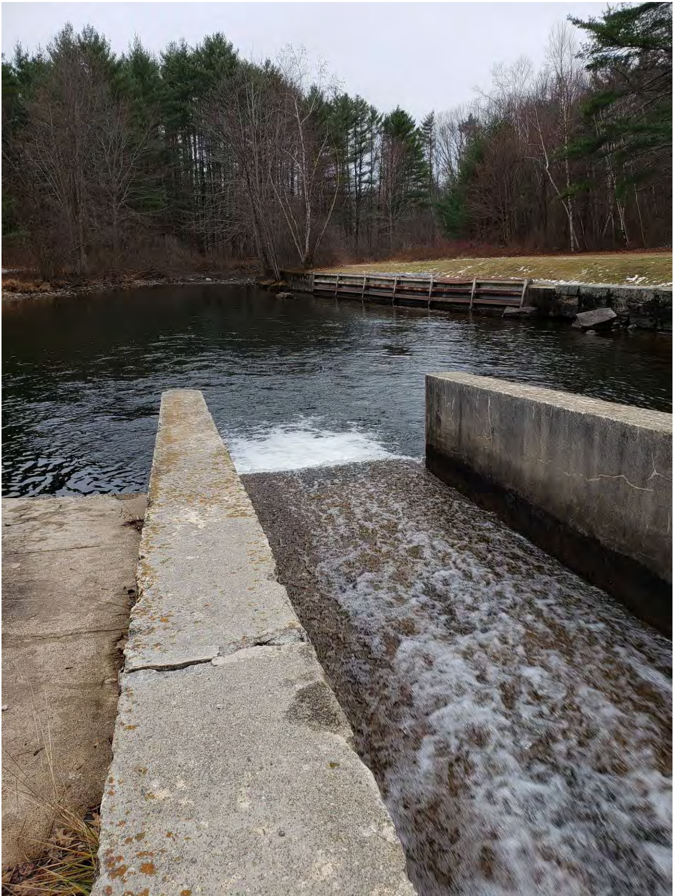
PHOTO 32: SLUICEWAY CHANNEL DOWNSTREAM OF GATE.
