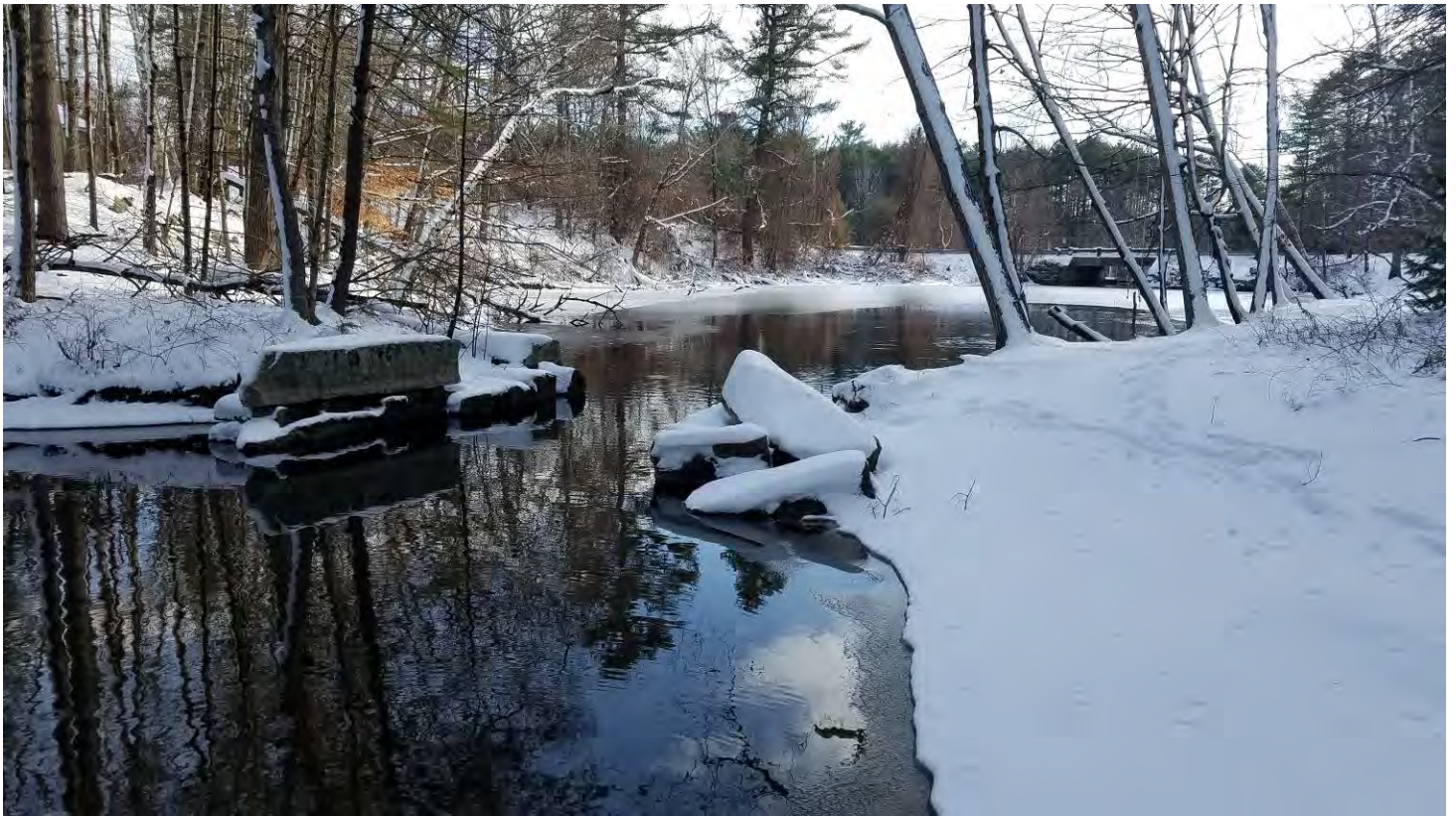
PHOTO 1: CONCRETE BLOCK STRUCTURE LOOKING BACK TOWARDS DAM.
