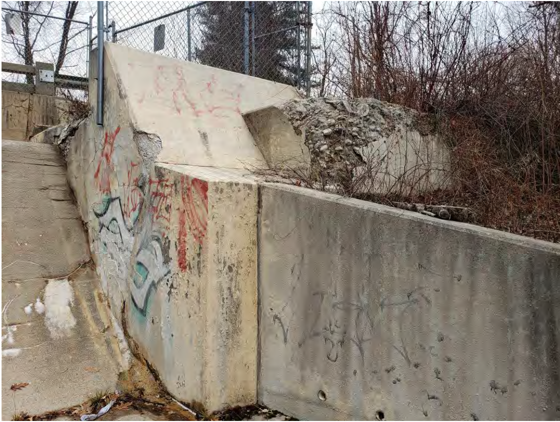
PHOTO 9: LEFT ABUTMENT CONCRETE RETAINING WALL.
