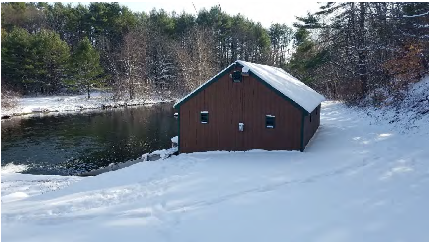
PHOTO 23: FISHWAY BUILDING AND ACCESS ROAD (UNDER SNOW COVER).
