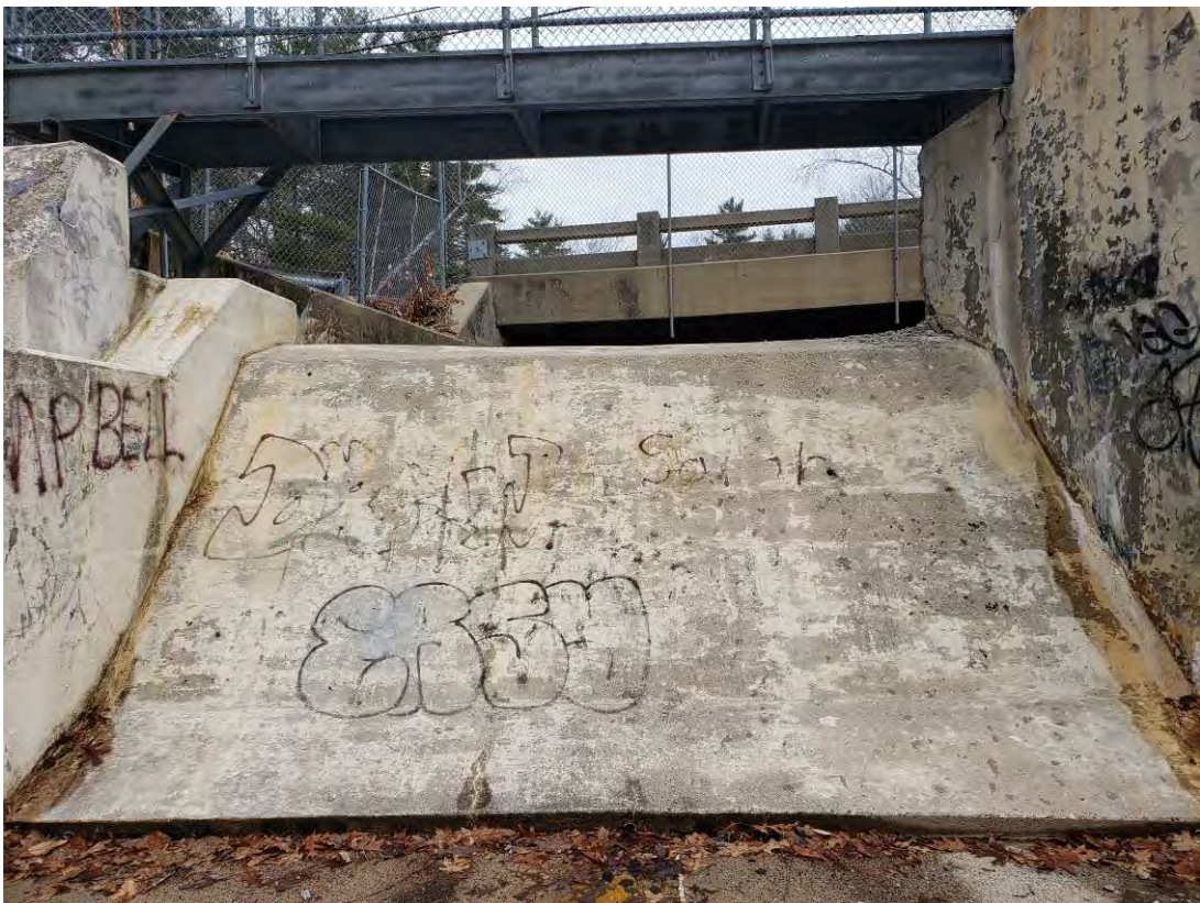
PHOTO 12: DOWNSTREAM FACE OF THE RIGHT OVERFLOW SPILLWAY.
