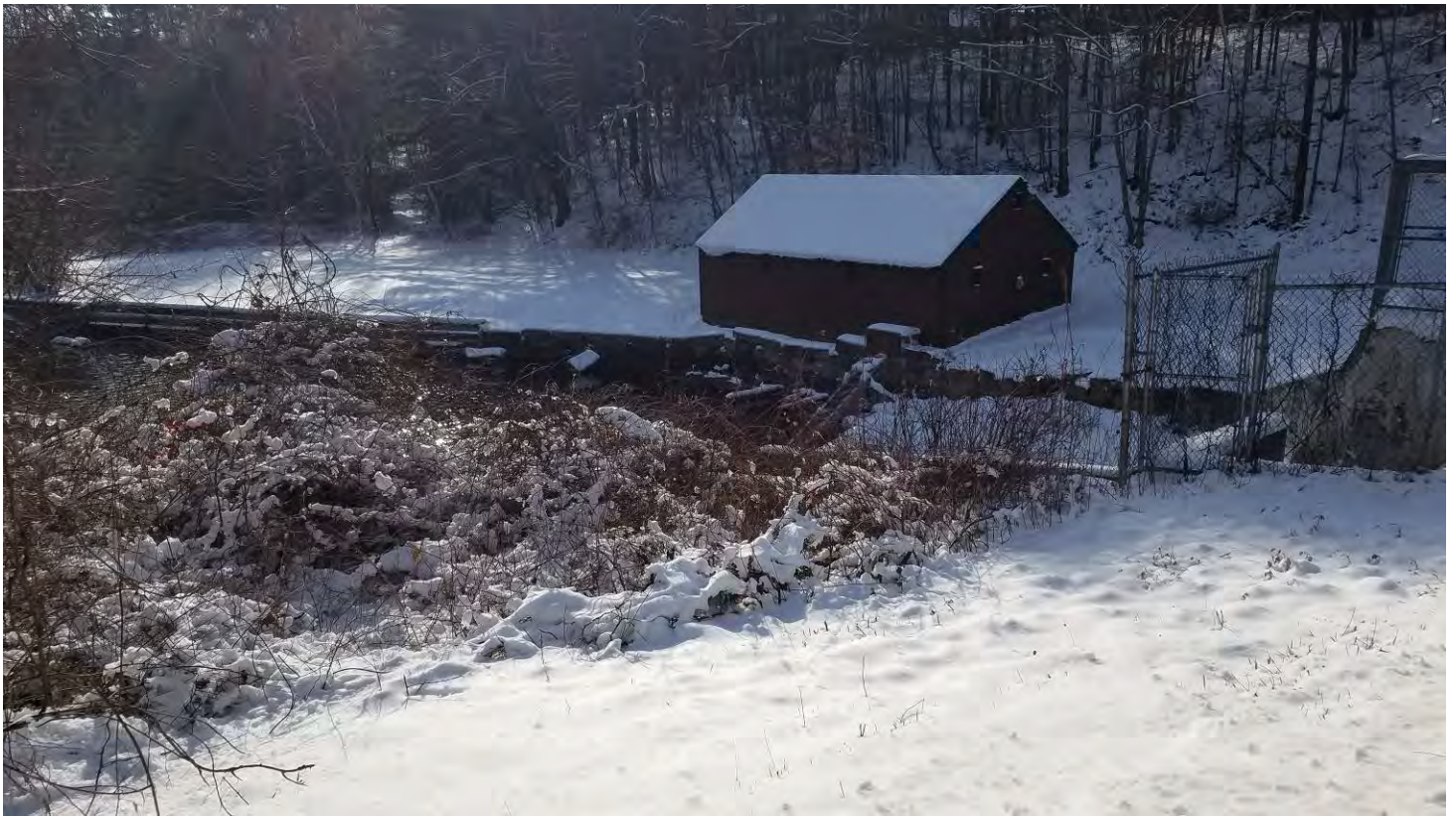
PHOTO 8: LEFT ABUTMENT EMBANKMENT DOWNSTREAM FACE.
