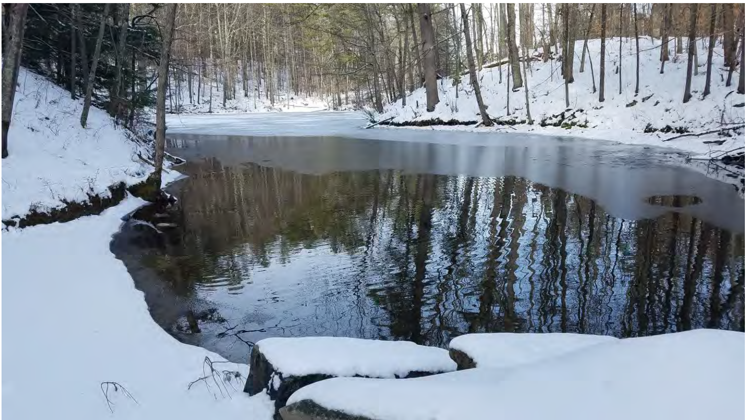
PHOTO 2: RESERVOIR UPSTREAM OF CONCRETE BLOCK STRUCTURE.
