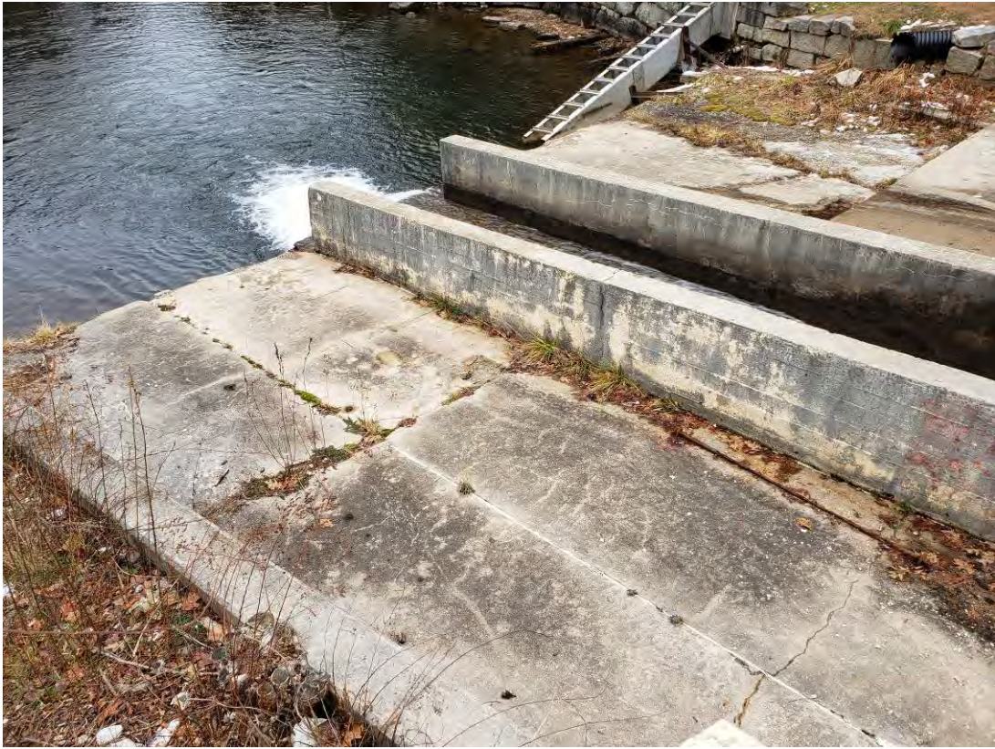
PHOTO 30: APRON DOWNSTREAM OF LEFT OVERFLOW SPILLWAY.
