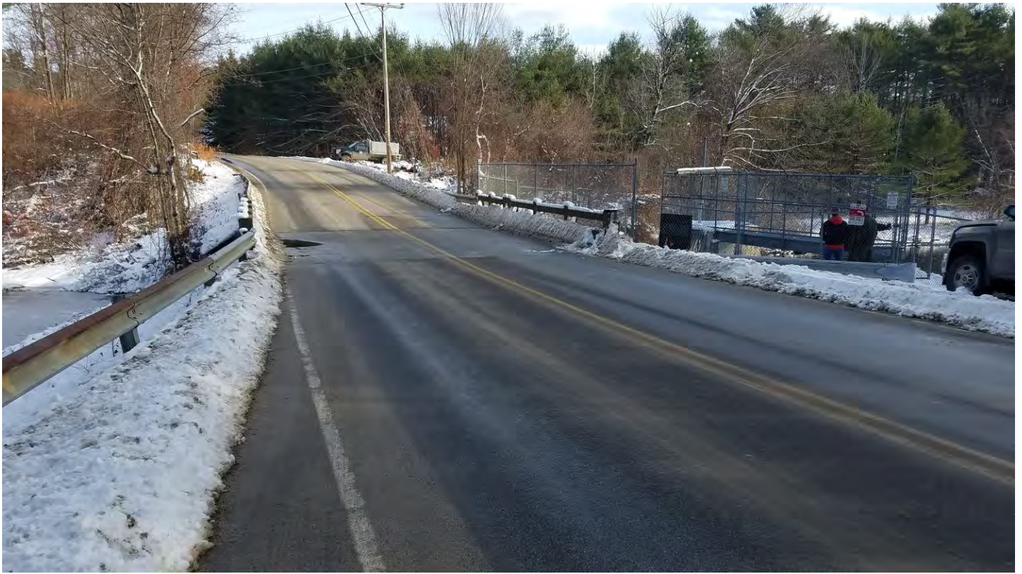
PHOTO 7: MILL STREET BRIDGE AND LEFT ABUTMENT.
