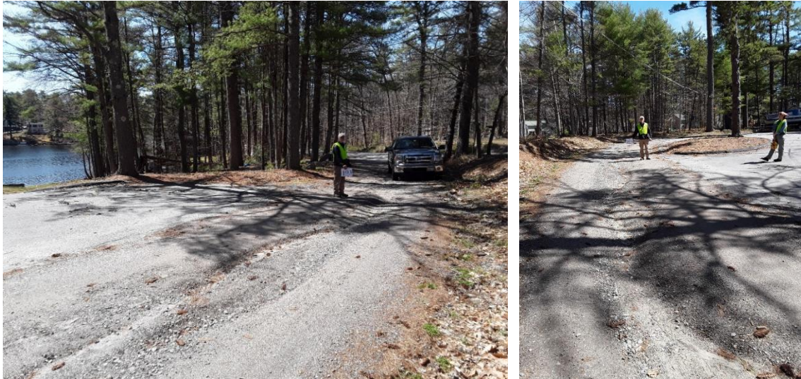
(Left) View down Haskell Ave, where a rill has formed within the unpaved road surface. (Right) View upslope of the rill.
