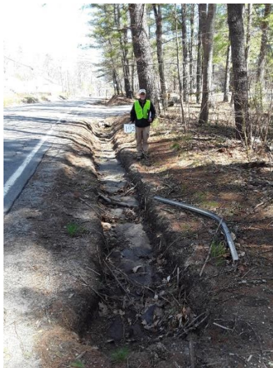
(Left) View of the start of the gully on the lakeside of Route 85, just south of Haskell Ave. Steep banks indicate severe gully ditch erosion. (Right) View of where the gully overtops onto the paved road shoulder, before veering towards an old detention basin above the lake.
