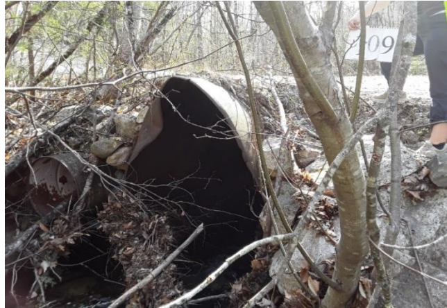
The culvert beneath the driveway, which is crushed.
