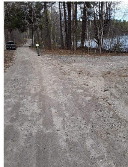
View down Kossow Lane. Erosion is occurring on both shoulders of the road.
