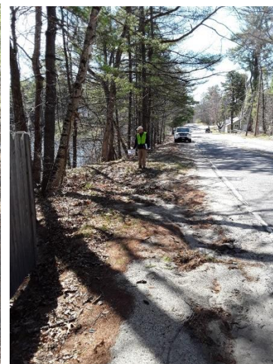
(Left) View of the start of the gully on the lakeside of Route 85, just south of Haskell Ave. Steep banks indicate severe gully ditch erosion. (Right) View of where the gully overtops onto the paved road shoulder, before veering towards an old detention basin above the lake.
