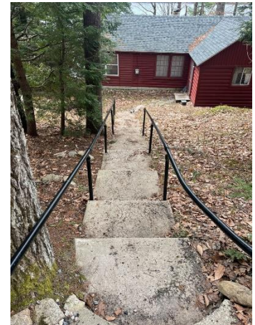
View looking down the top set of stairs from Mawaga Road. Signs of erosion are present at the staircase bottom.
