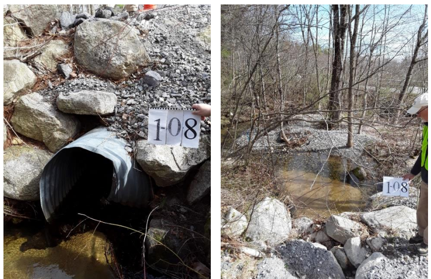
(Left) The culvert beneath Davis Brook Road is rusting and undercutting the bank.
