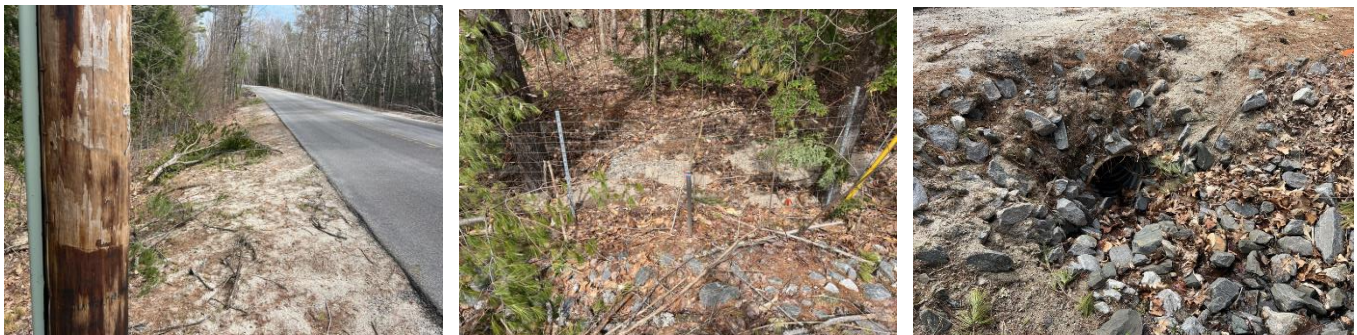
(Left) View of the roadside, where sediment washes. (Center) View of the land downslope of the roadside, where sediment deposition is evident. (Right) View of the small culvert downslope of the road.
