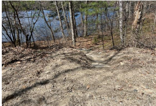
Sediment from Rosewood Drive washed down onto steps providing access to the lake.
