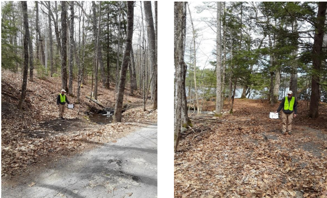
(Left) View of the location where the stream overtops onto Myron Hall Road, causing erosion of the road.
