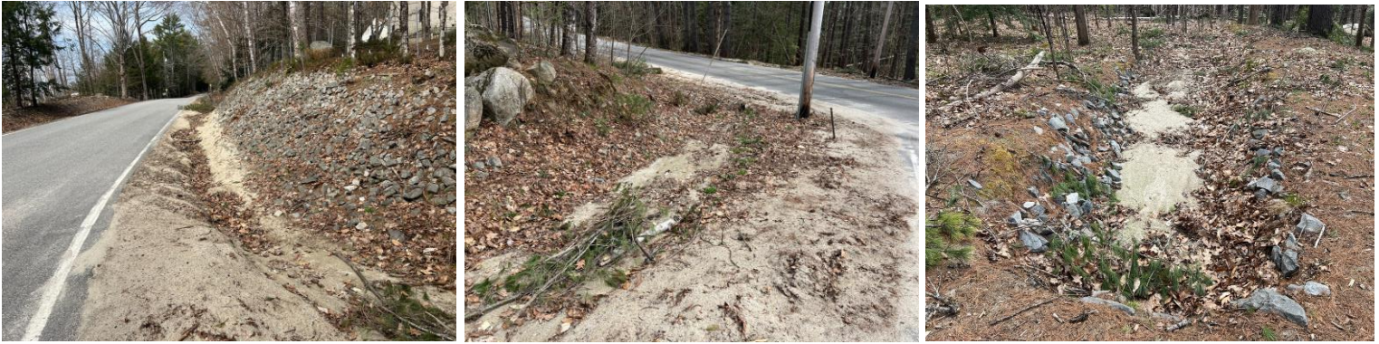
(Left) View up Mountain Road where roadside erosion is evident. (Center) View down Mountain Road towards the intersection with Conesca Road. (Right) View downslope of the intersection of Mountain Road and Conesca Road, where runoff has deposited sediment.
