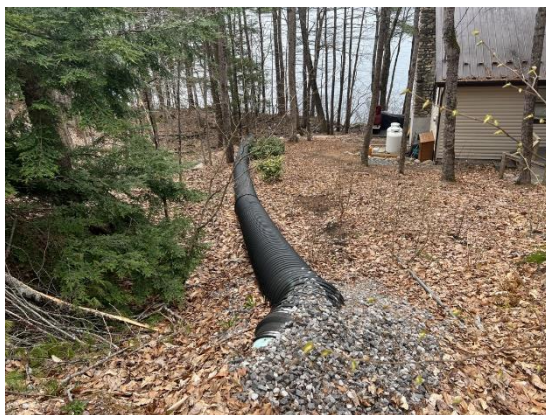
(Left) View looking down the plastic "culvert" towards the lake. (Right) The inlet of the culvert before it passes beneath Mawaga Drive.
