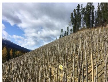
Left: How to harvest a live stake. Upper: Storage of live stakes for later use. Lower: Live stakes installed on a slope.
