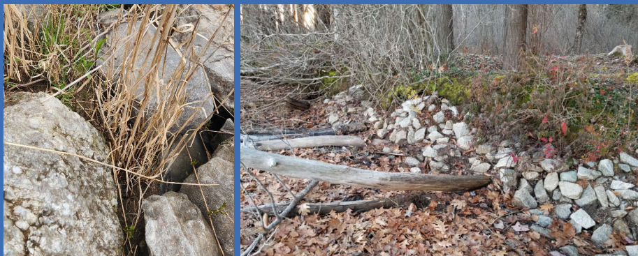
Rooted riprap has soil between the rocks and no plastic geotextile underneath, allowing plants to grow deep roots that help to stabilize the shore.
