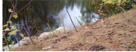
Live stakes installed on a shoreland slope.
