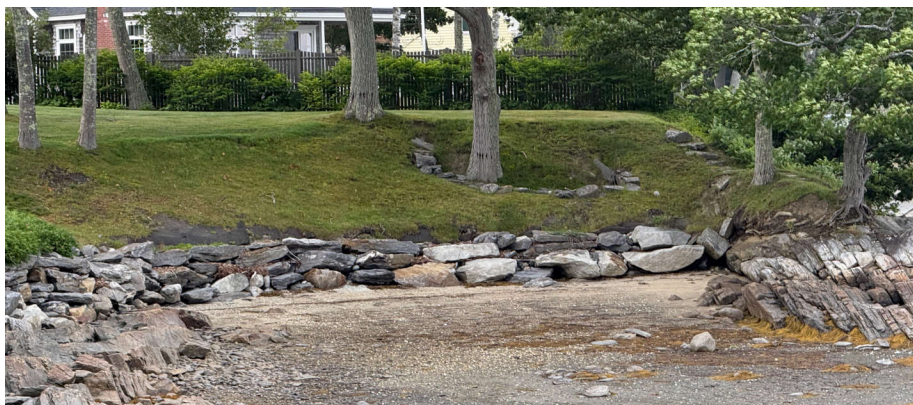
Example of a shore with riprap and sparse shrubs and trees. Planting a dense mix of shrubs and trees could reduce erosion and improve wildlife habitat. (P. Taylor/Waterview)
