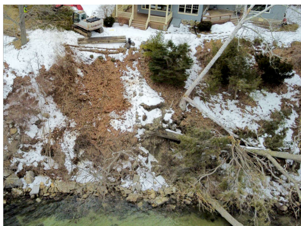
Treefall contributed to instability and erosion of this high, steep slope. (Linkel)
