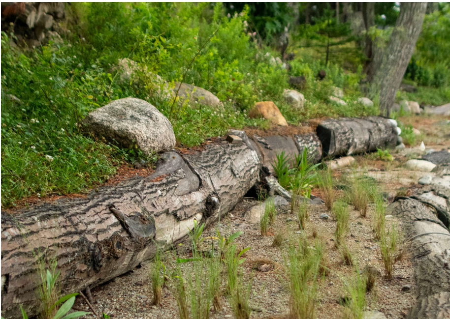
This shoreline was stabilized using logs and dense vegetation. Existing vegetation was retained, and new plants were added. (The Home Place Team)
