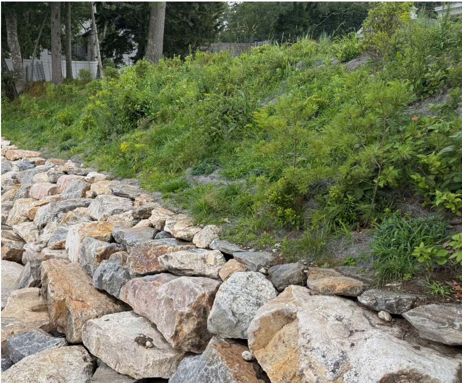
A newly installed stabilization project that was designed to repair and protect a shoreline heavily damaged by storm waves in prior years. The riprap was installed during winter, the plantings were added in the spring, and this photograph was taken in the summer. (P. Taylor/Waterview)
